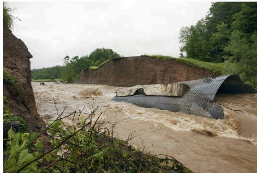
Figure 14A. Top—Collapse of Interstate Route 88 over Carrs Creek near Unadilla (Exit 10), NY, on June 28, 2006. Bottom—Carrs Creek and washed-out culvert at Interstate Route 88 near Unadilla (exit 10), NY, on June 28, 2006. Photos courtesy of The Daily Star, taken by staff photographer Julie Lewis.
